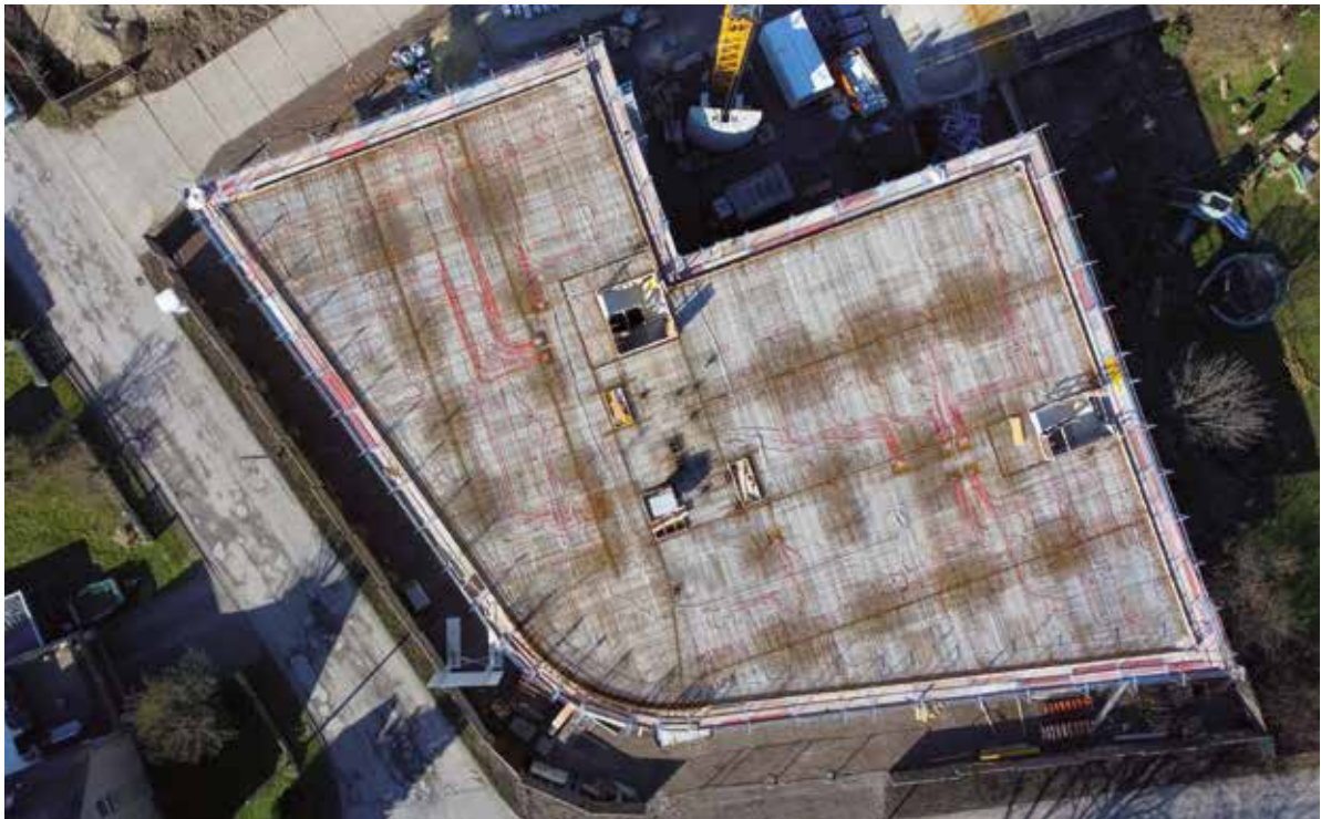
© Heitfeld Baugesellschaft mbH
